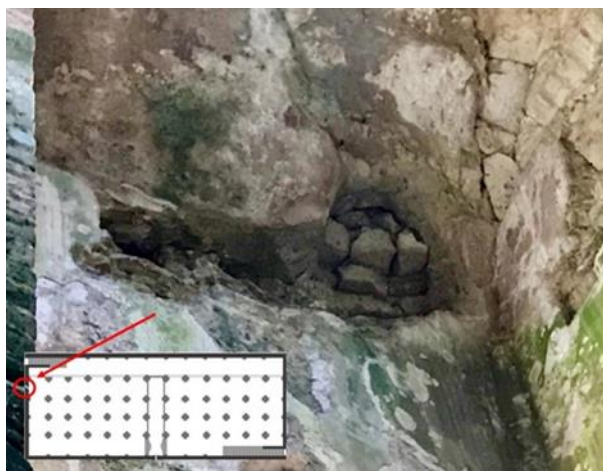
Photograph 16 Probable Aqueduct entry on right - note arched top
