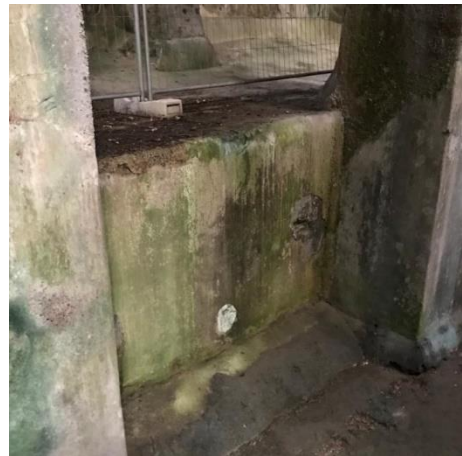
Photograph 20 The small, blocked, possible outlet at the north end of the central basin
