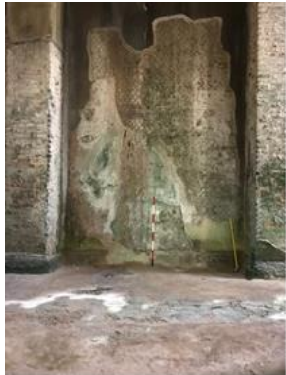
Photograph 12 Wall between two side buttresses
