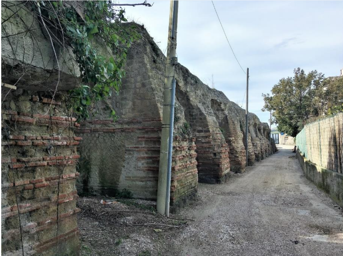
Photograph 6 Supporting buttresses on the external NE wall
