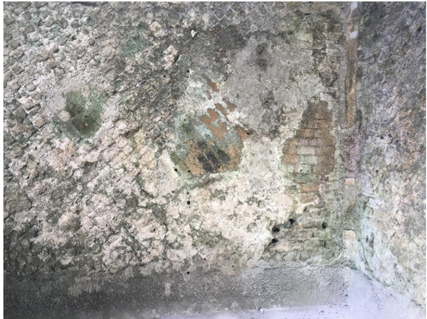
Photograph 21 Corner of internal SE wall showing repair work
