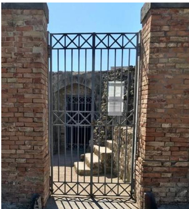
Photograph 3 Visitor entrance at the NW corner with entrance to Piscina in the background
